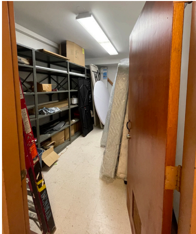
Typical Storage Closet
